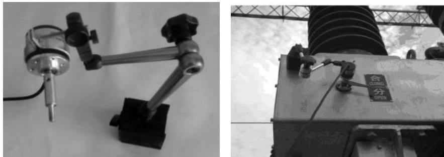
Figure 10: 35KV SF6 switch sensor installation
